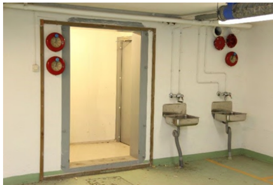
Figure 15: Water points are visible next to the entrance to the civil defense shelter, as well as ribbing around it for the construction of a lock tent. The lock tent serves as a vestibule for the shelter.
