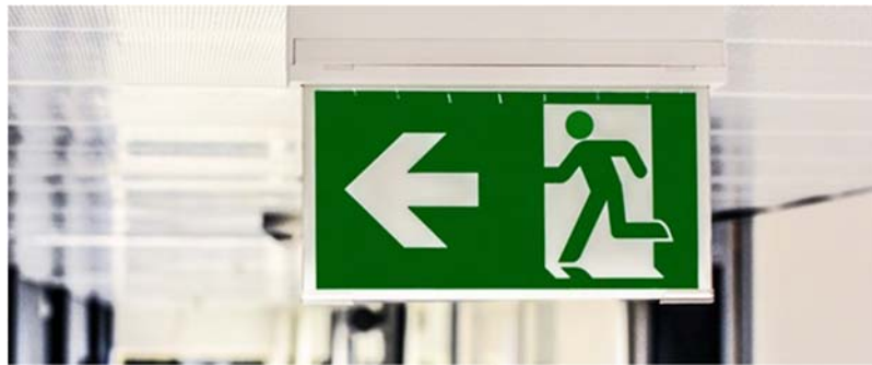
Figure 19: Escape route sign.
