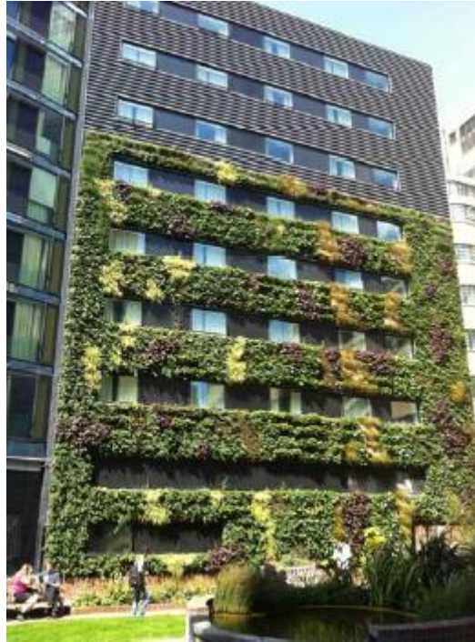
Green wall Tower Gateway, Londra. Fonte: https://assets.publishing.service.gov.uk (Gary Grant)
