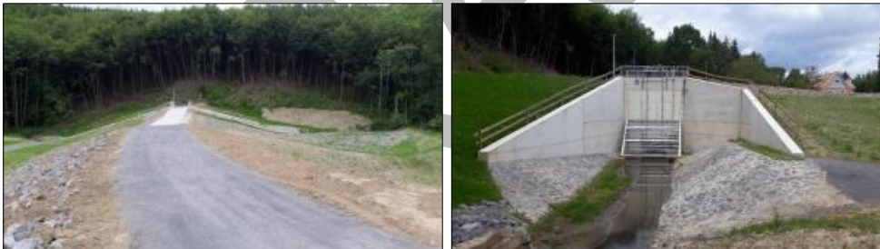
Figure 11: Example of a rainwater retention basin consisting of an earth dam with a passable and controllable throttle structure with associated measuring and control technology (the origin of the photo: GDV/VdS3521)
