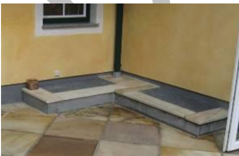
Figure 15: Examples of upstands for constructional openings (origin of the photos: GDV/EPZ)
