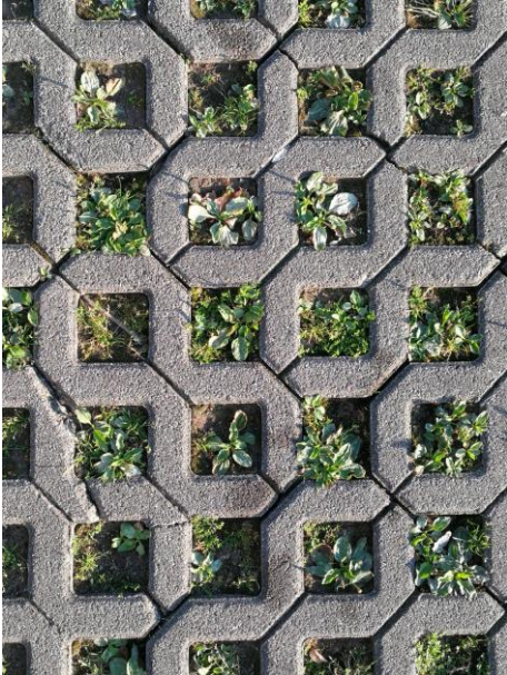
Figure 10: Example of water permeable ground fixing (the origin of the photo: Mingyi Wang)
