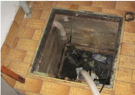
Figure 16: Examples of a pump shaft (origin of the photos: EPZ)
