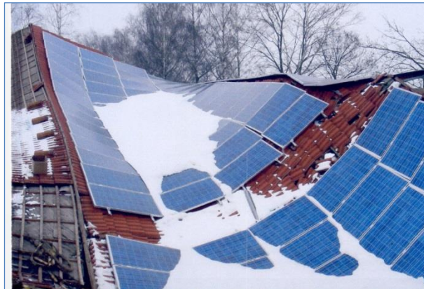
Figure 2 A roof with PV modules collapsed under snow load (source: VdS 3145)
