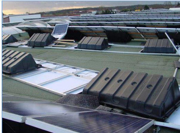
Figure 1 Example of storm damaged PV modules on the roof (source: VdS 3145)
