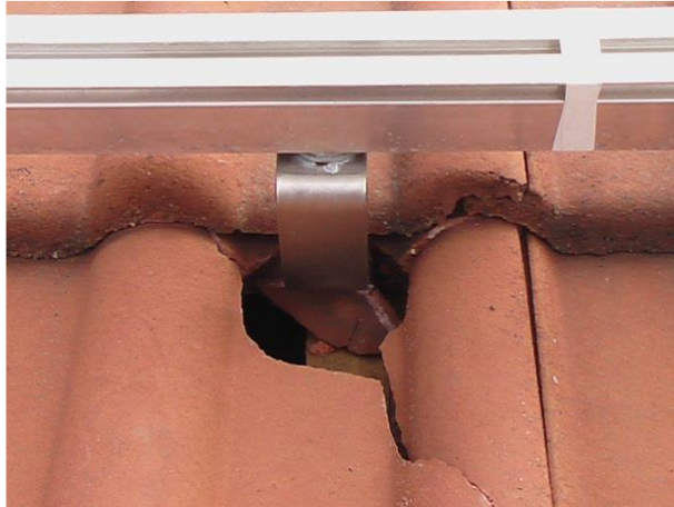
Figure 4 A roof tile damaged by roof hooks for attachment of PV modules (source: VdS 3145)
