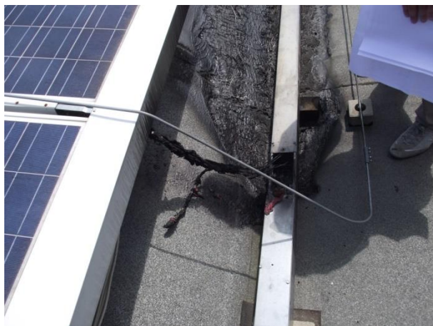
Figure 5 Damage on roof covering caused by fire of PV-installation (source: Guido G. Zaccarelli)
