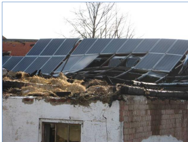
Figure 3 Fire damaged roof with destroyed PV modules (source: VKB)
