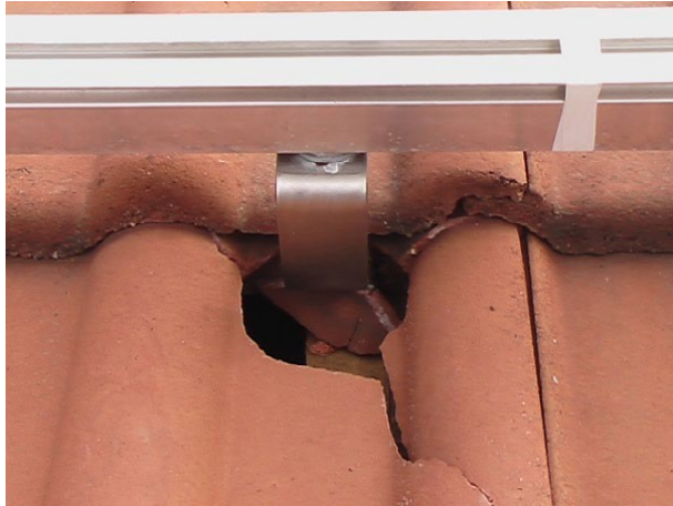
Figure 7 A roof tile damaged by roof hooks for attachment of PV modules (source: VdS 3145)
