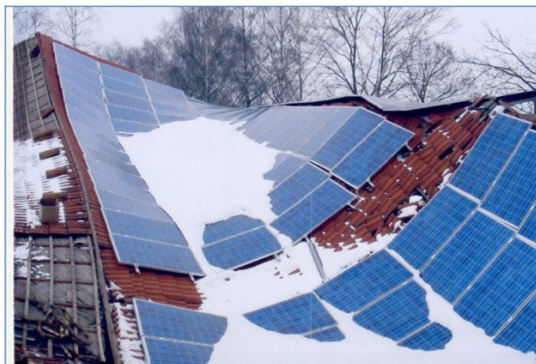
Figure 5 A roof with PV modules collapsed under snow load (source: VdS 3145)
