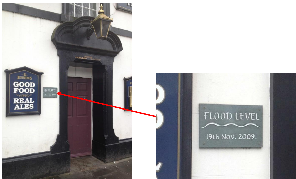
Figure 2: Flooding can have a severe and prolonged impact on both small and large business operations
