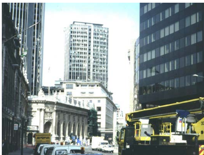
Figure 3: The company occupying the tower block, which was severely damaged by a vehicle bomb, was back in business in alternative premises within 48 hours thanks to an effective contingency plan
